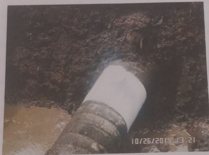
REPAIR WAS DONE BY CONNING.
